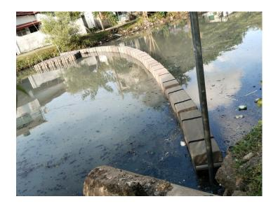
INSEE Ecocycle engineers have utilized environmentally friendly practices to fabricate these ocean strainers internally by incorporating scrap materials collected from waste management operations and cement production.
