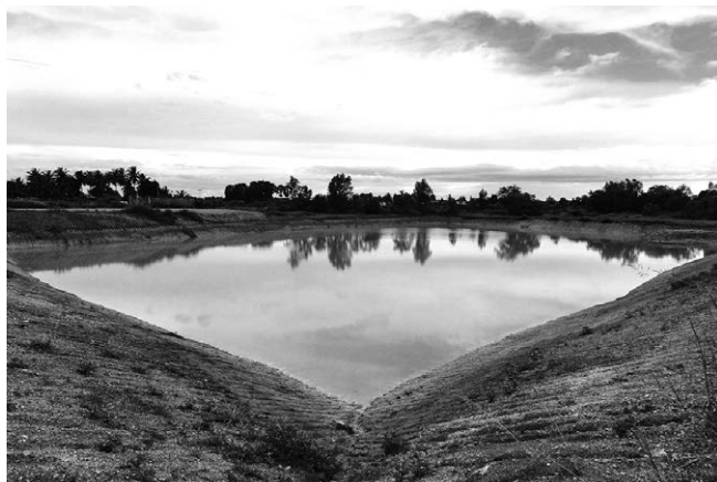
Figure 2: Second freshwater pond (at first stage with capacity of about 35,000m 3 )
