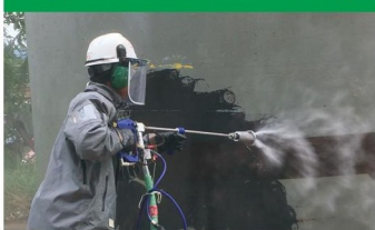
High Pressure Water Jetting
